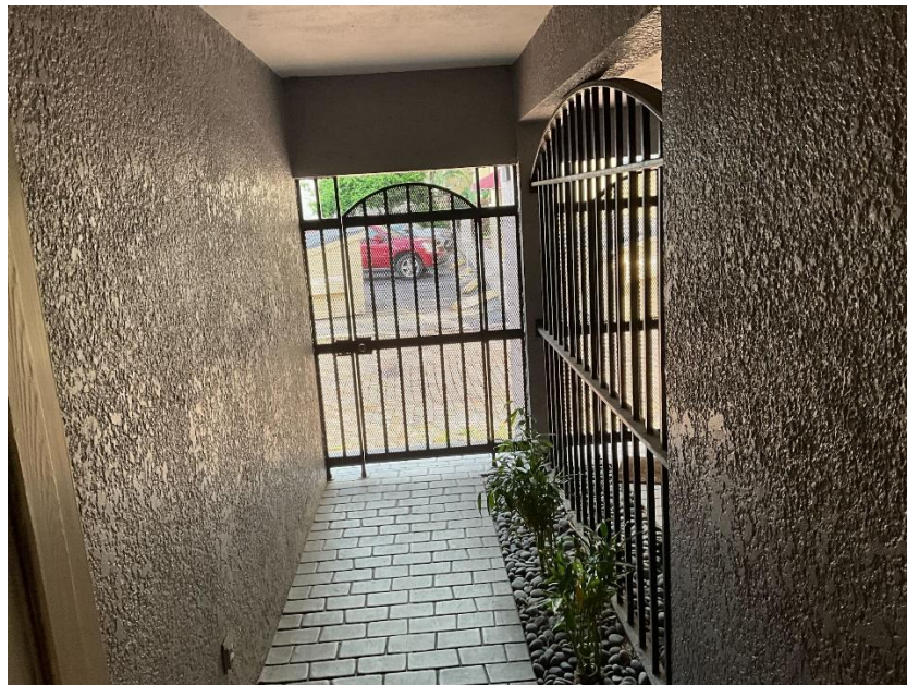
14. View of the walkways in the habitable areas of the building.
