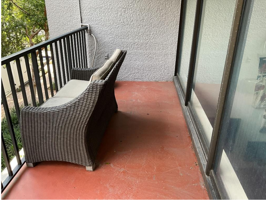
15. View of the balcony of the habitable areas of the building.
