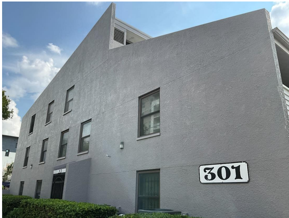
18. Side view of the exterior of the building.
