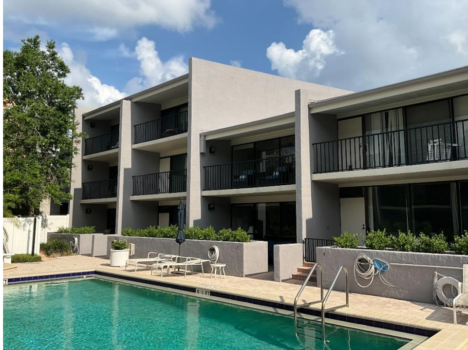
17. View of the exterior of the building.
