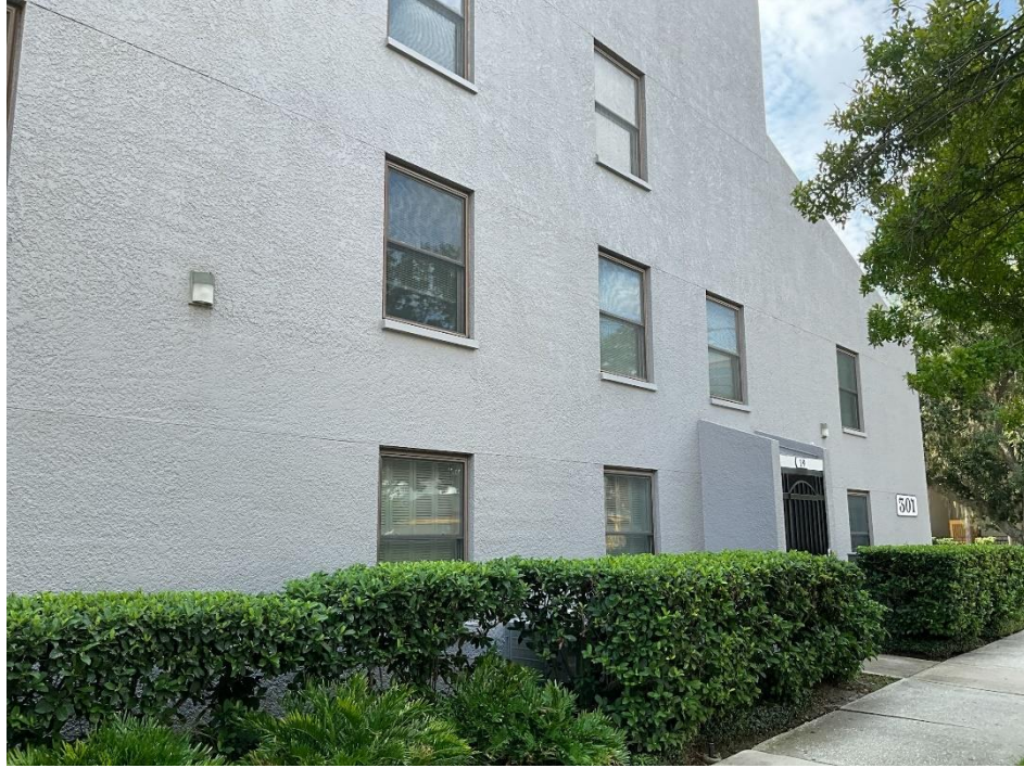
7. View of the stucco on the side of the building.
