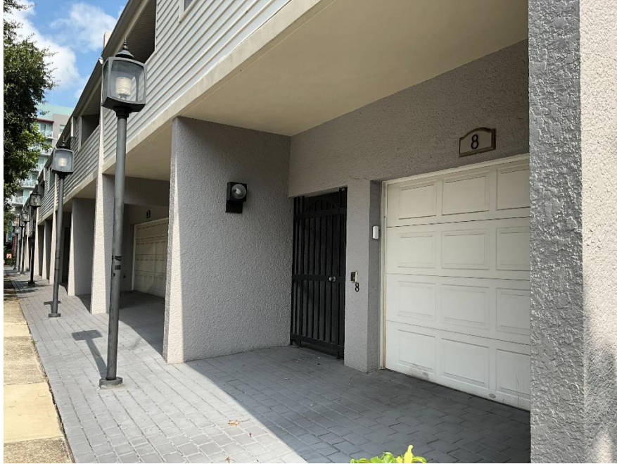
3. View of the garage and siding of the building.
