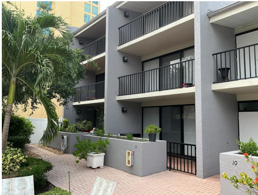
2. Front view of the subject complex (facing the pool).
