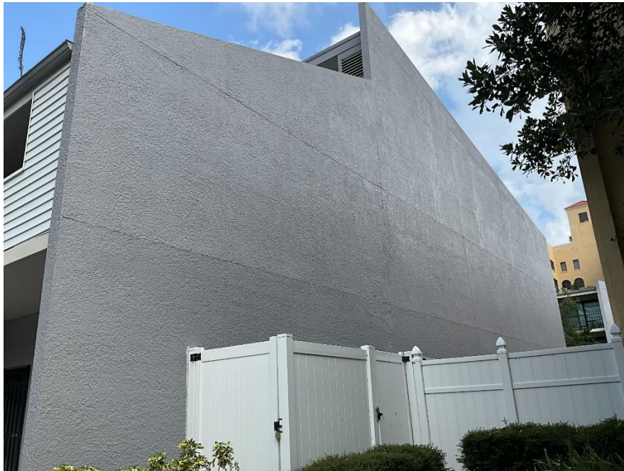
4. View of the stucco on the side of the building.
