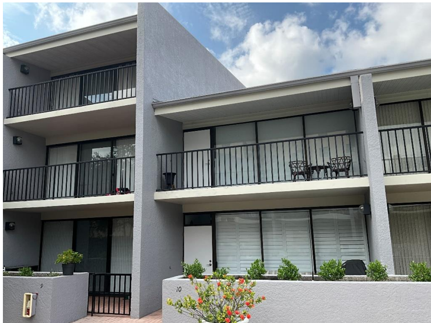
16. View of the exterior of the building.
